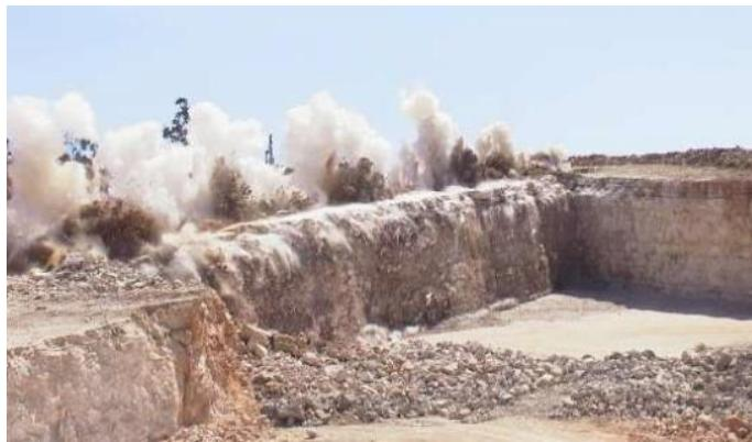
*Figure 10 - Application of explosives in quarries.*
