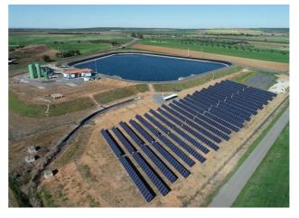
Efacec. Thermographic and visual inspection of all equipment in this plant was carried out, in addition to the plotting of I-V curves of the photovoltaic sets and solar tracking tests.
